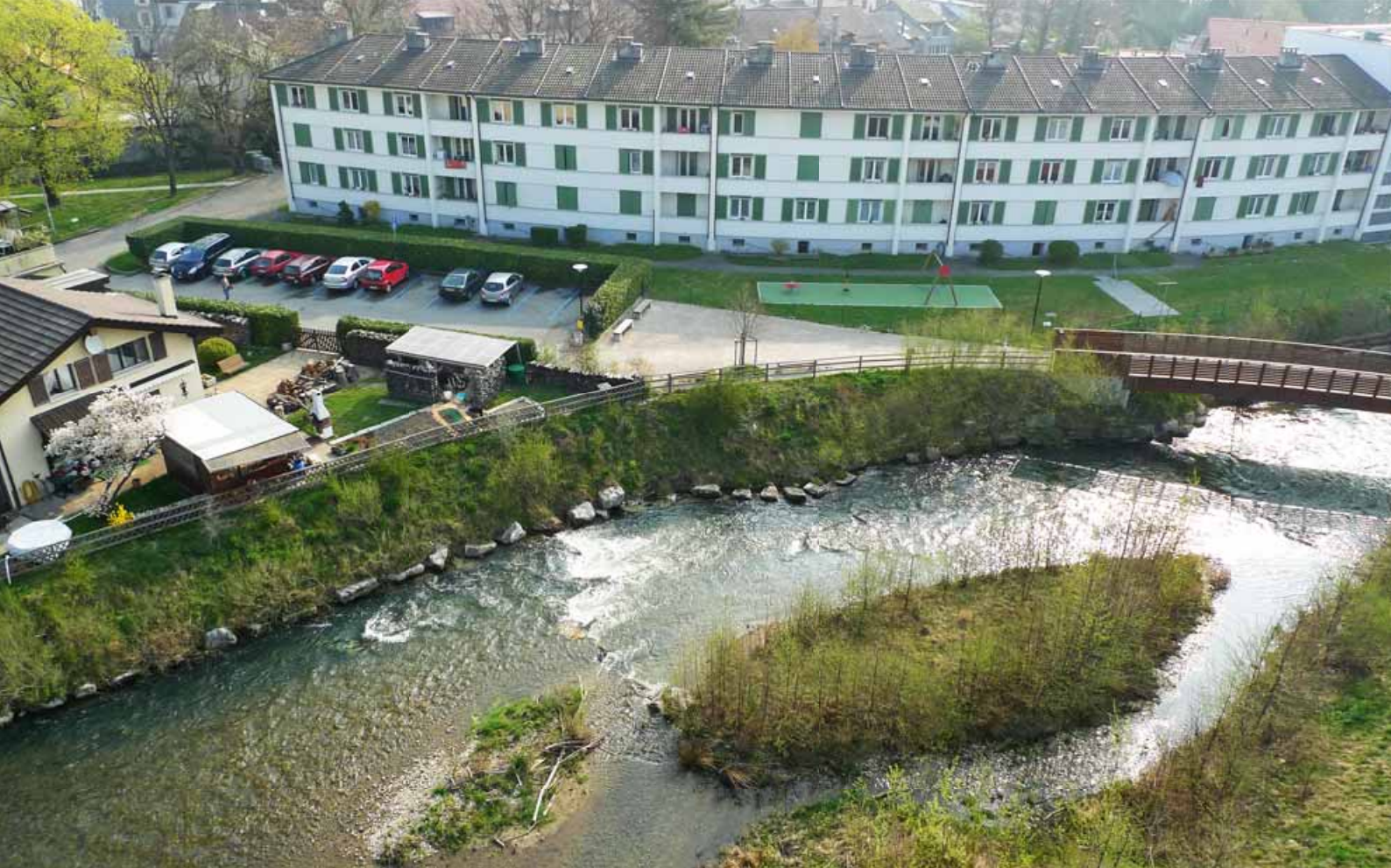
Upgrading in populated areas: the successful revitalisation of the Versoix River (GE) is the result of careful planning.
