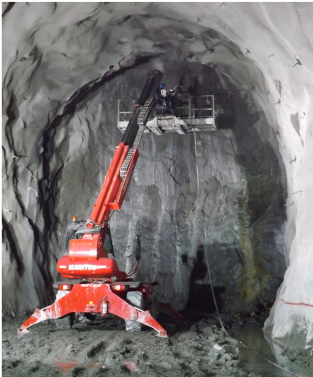
Figure 2: Progress of excavation of more than 10 m high headrace tunnel, performed by drill and blast.
