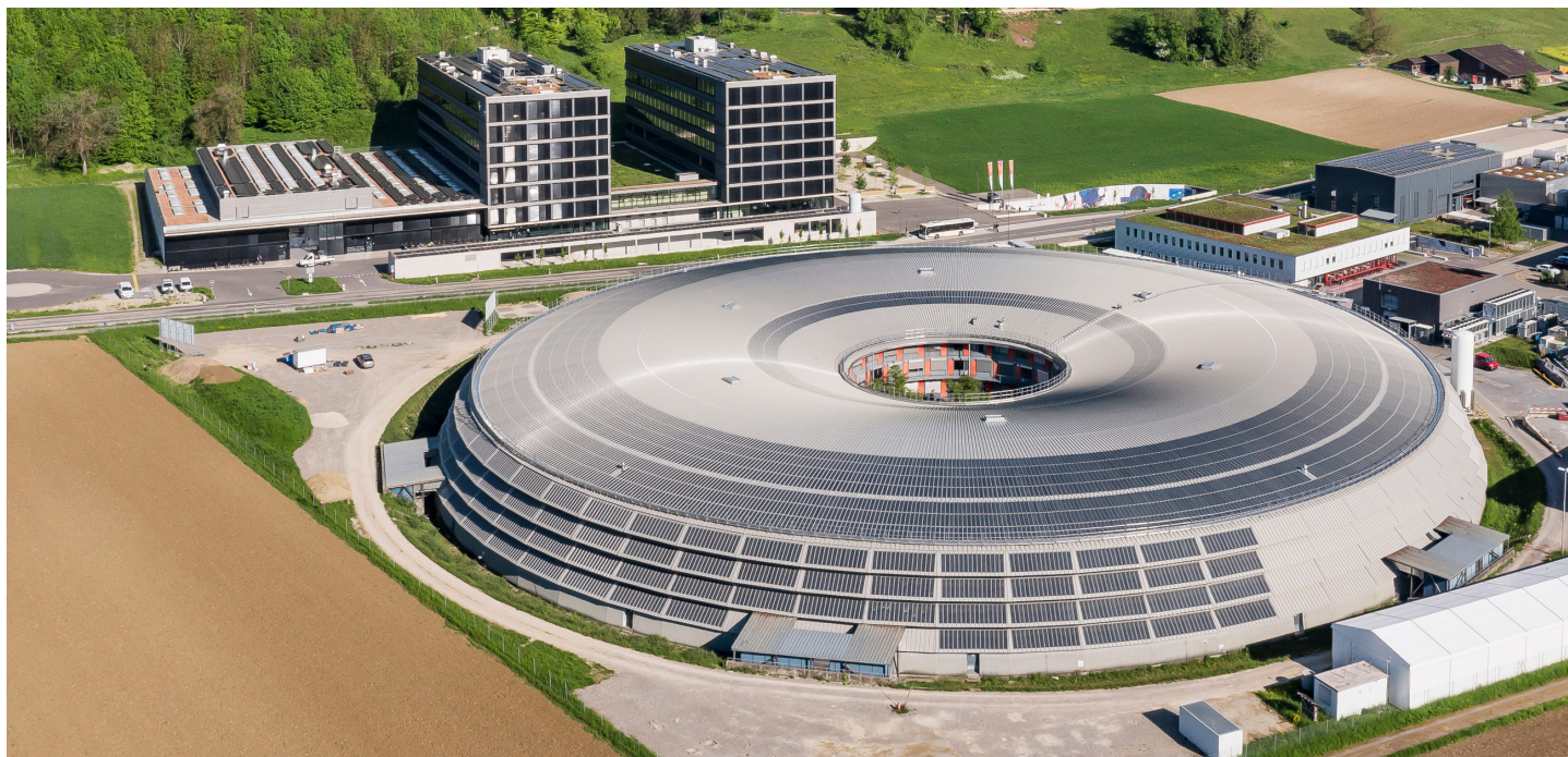
Figure 1. The renovated SLS building housing now SLS 2.0, showing the new aluminium roof fitted with solar panels.
