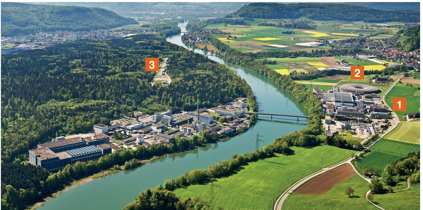
Fig. 6: The PSI campus consisting of the former SIN (west bank) and EIR (east bank). 1: SINQ, 2: SLS, 3: SwissFEL
