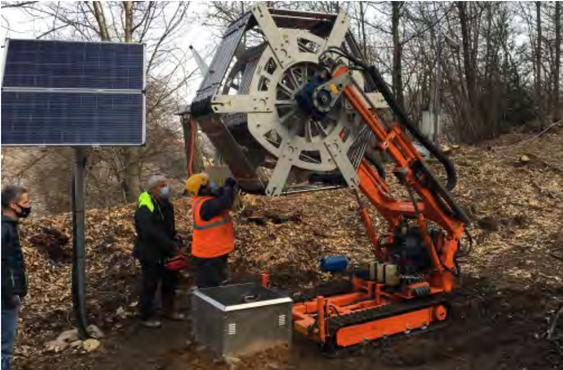
Figure 2. On-situ installation of the DMS column
