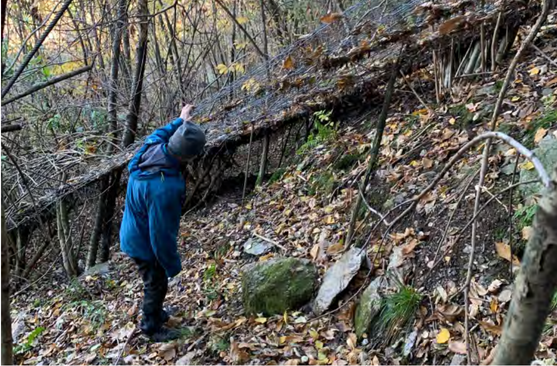
Figure 1. Net in adherence stretched by the movement of the slope
