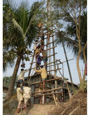
Figure 3. Construction of an arsenic-safe deep tubewell.
