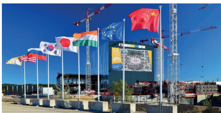
Figure 2: The ITER construction site (with the 60-meter-high tokamak assembly hall). © ITER
