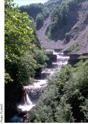
Structural measure to pre flood-related dam Durnagelbach, Gl
