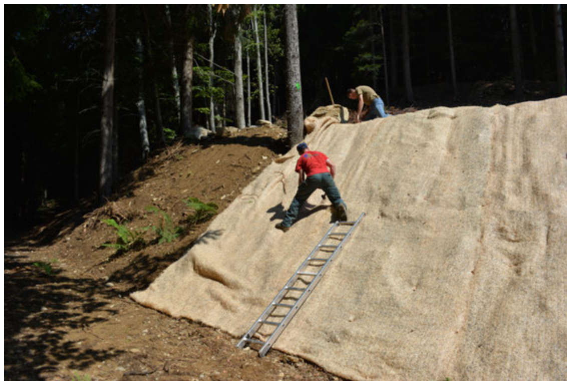
Figure 1. Installation of the Wood Wool mats on a test site in Gramiröi (Val Leventina, Canton Ticino).
