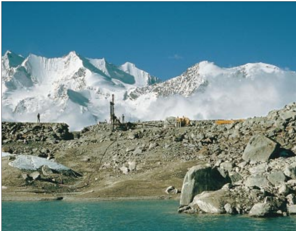
Photo 6.3: The injection drillings on the dam at Lake 1 protect the moraine against further erosion and prevent an outburst of this lowest-laying lake. The Dom and Lenzspitze mountains are in the background. (Photo: A. Kääh, University of Zurich)
