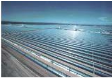
KJC, Kramer Junction, USA
