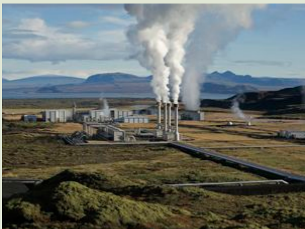
Geothermal power plant in Iceland.
