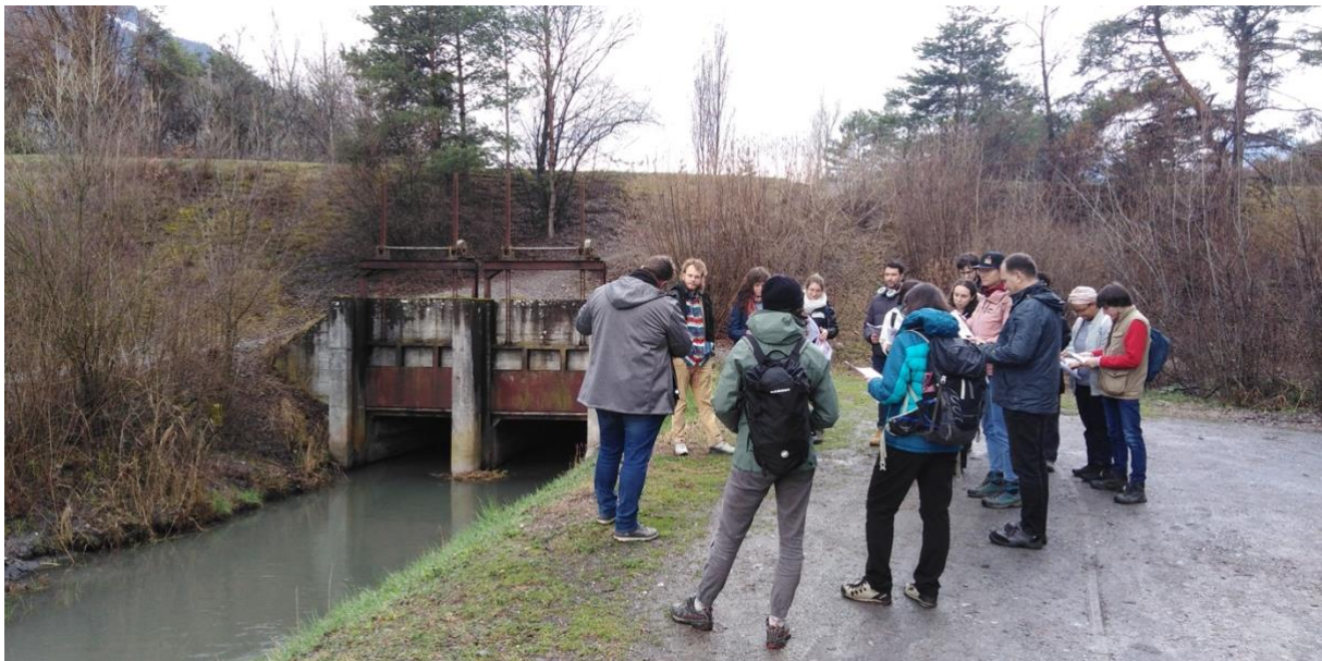
The Sion-Riddes canal, crossing the Lizerne River: an enlargement of the tunnel is planned to avoid the accumulation of water against the Lizerne dam in the event of the Rhone overflowing its bed. Photo: J. Bussard, 24 March 2023
