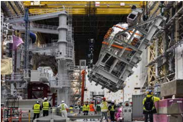
Moving upright a 440 t sector of the vacuum vessel, to bring it to the assembling tool on the left of the image (Korean sector, 11.12.2021). © ITER.
