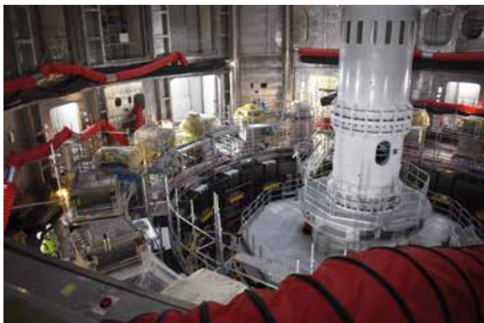
Inside the tokamak pit, assembling the tokamak components. © AP
