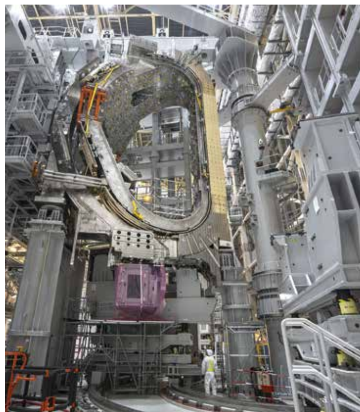
The first sector of the vacuum vessel (out of 9, 440 t) mounted on the assembly tool, surrounded by its 2 TF coils (2 x 320 t). © ITER
